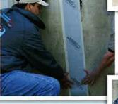
Finishing the Techni-Crack\* membrane with sealant.
