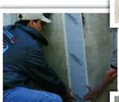
We apply hydrophobic gel on the back of the Techni-Crack\* membrane and apply it to the wall. We then tie it into the Water Trek Aqua Route" system or drywell.
