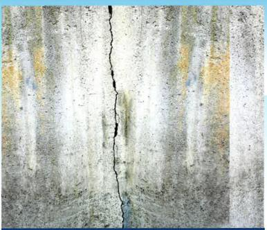
Poured foundation wall cracks generate water onto the basement floor.
