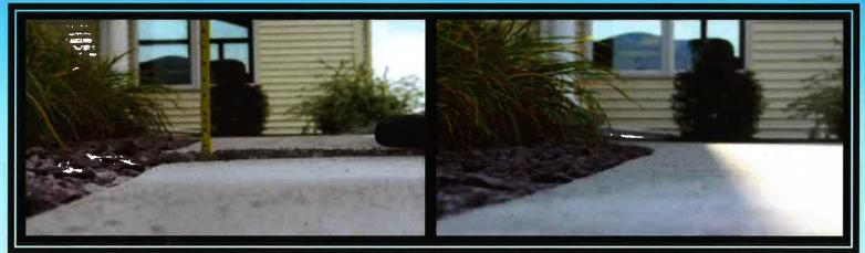
Call it mud-jacking, slab-jacking, grout injection or simply concrete lifting – they are one in the same. Whatever the case, the process entails drilling small holes through the concrete of affected areas and pumping cement grout underneath. As the mixture flows beneath the surface, voids and depressions are filled and the concrete is raised to the desired height.
