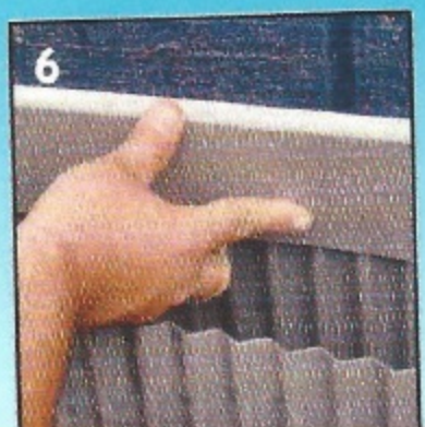
6 7 A SPECIAL "COVER PIECE" IS INSTALLED OVER THE TRENCH PROTECTOR STOPPING WATER FROM GETTING TO THE SILL PLATE.
