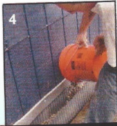
4 5 STONE IS BACKFILLED INTO THE CURTAIN DRAIN™ SYSTEM. GREY IS THE STANDARD COLOR USED, BUT WHITE OR OTHER COLORS CAN BE SUBSTITUTED UPON REQUEST.
