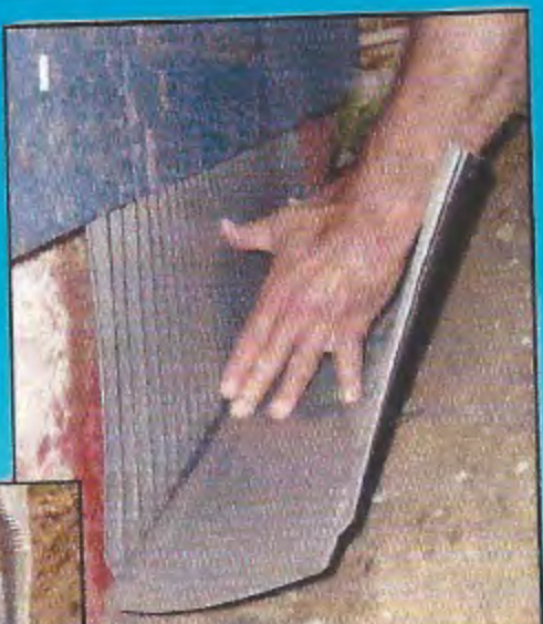
1 A TRENCH IS DUG IN THE EFFECTED AREA WHERE WE INSTALL OUR DOUBLE "CURTAIN DRAIN™" PROTECTOR TO STOP DIRT FROM CLOGGING OUR WATER TREK AQUA ROUTE® CONDUIT.
