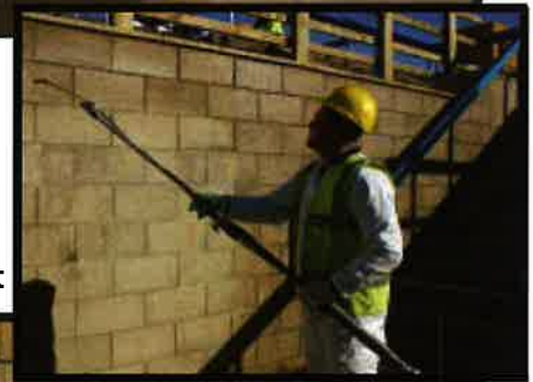
Concrete wall before, during and after PaviX treatment
