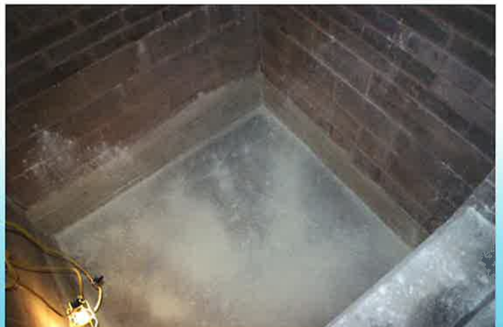
Elevator pit after Sofix® 700 and CCC 150 treatment
