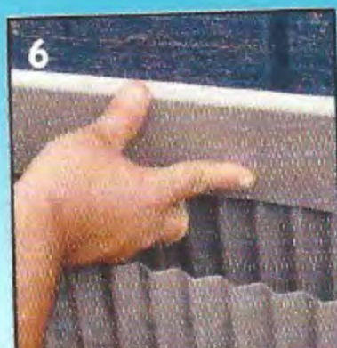
6 7 A SPECIAL "COVER PIECE" IS INSTALLED OVER THE TRENCH PROTECTOR STOPPING WATER FROM GETTING TO THE SILL PLATE.
