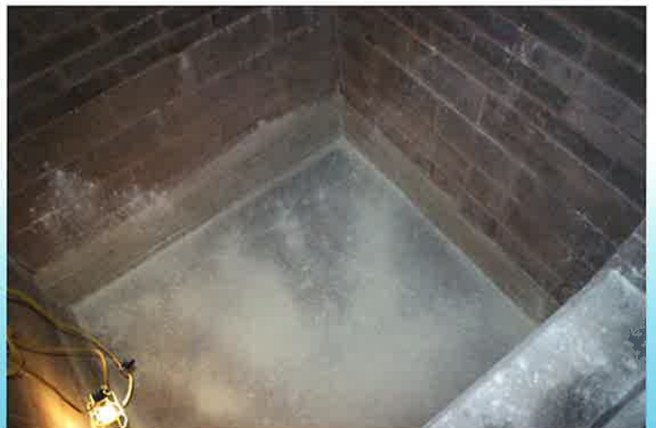
Elevator pit after Sofix ® 700 and CCC 150 treatment
