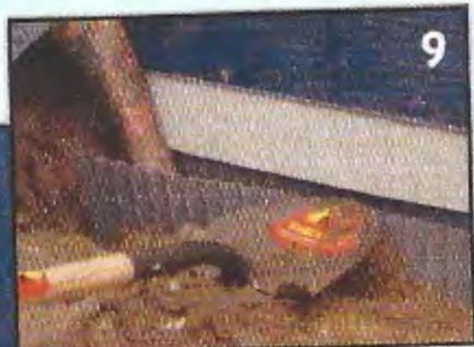
6 7 A SPECIAL "COVER PIECE" IS INSTALLED OVER THE TRENCH PROTECTOR STOPPING WATER FROM GETTING TO THE SILL PLATE.
