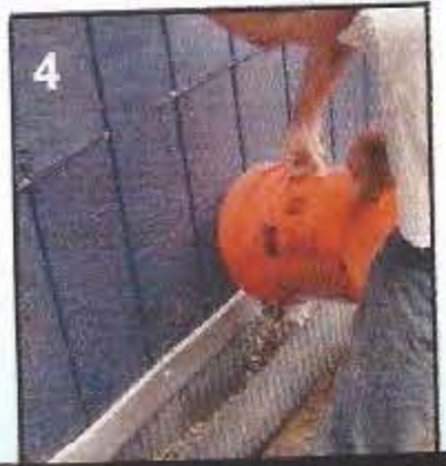
4 STONE IS BACKFILLED INTO THE CURTAIN DRAIN™ SYSTEM. GREY IS THE STANDARD COLOR USED, BUT WHITE OR OTHER COLORS CAN BE SUBSTITUTED UPON REQUEST.
