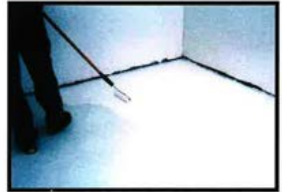
Damp proof treatment for concrete slabs.
