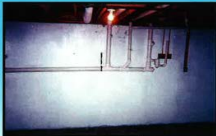
Interior masonry coating spray applied.
