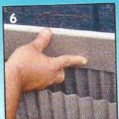
6 A SPECIAL "COVER PIECE" IS INSTALLED OVER THE TRENCH PROTECTOR STOPPING WATER FROM GETTING TO THE SILL PLATE.
