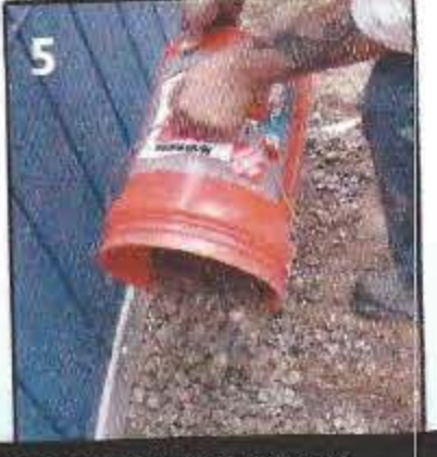
4 STONE IS BACKFILLED INTO THE CURTAIN DRAIN™ SYSTEM. GREY IS THE STANDARD COLOR USED, BUT WHITE OR OTHER COLORS CAN BE SUBSTITUTED UPON REQUEST.
