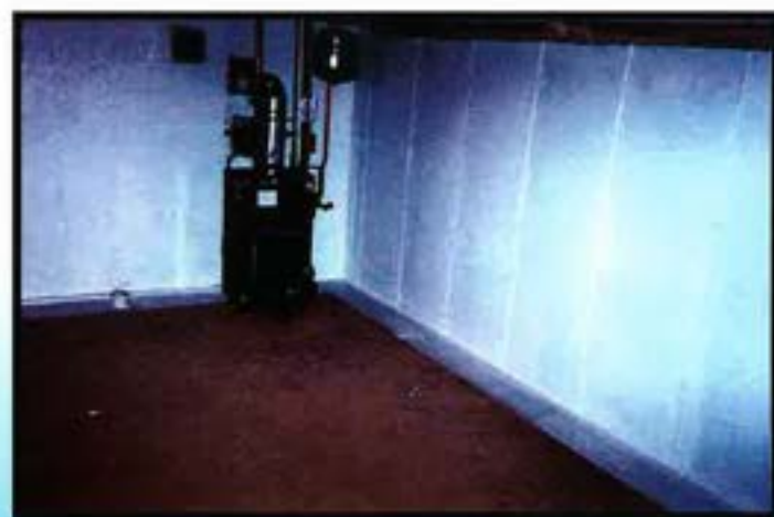
Sealed basement walls used with Water Trek system on floor.
